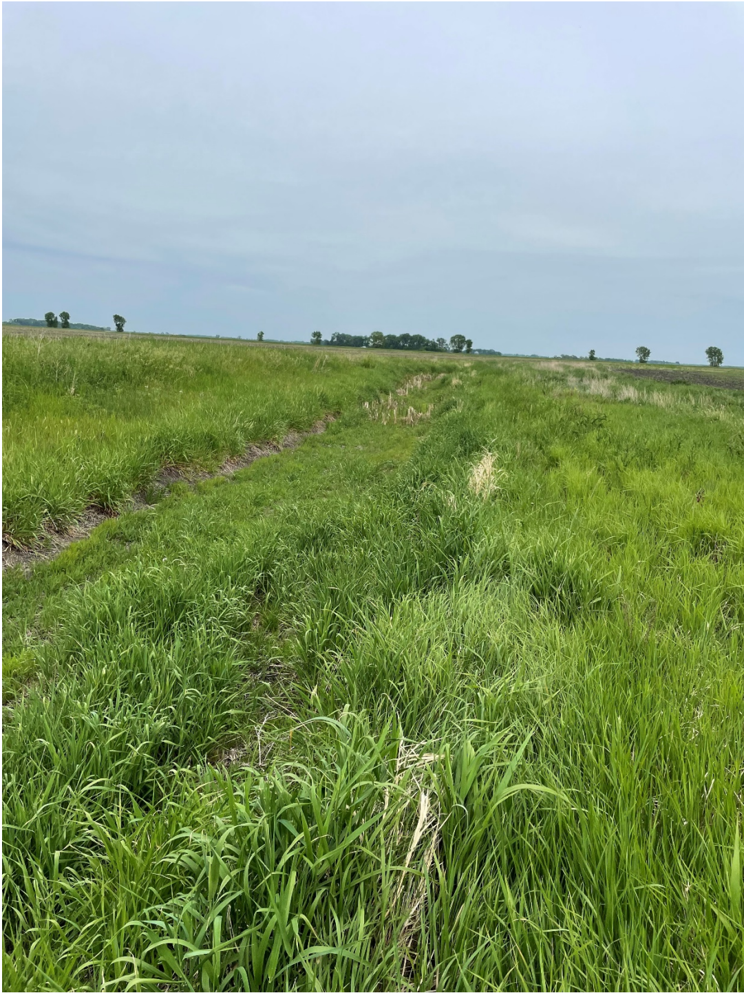
Example of an overgrown portion of the ditch. System needs cleaning in select locations.
