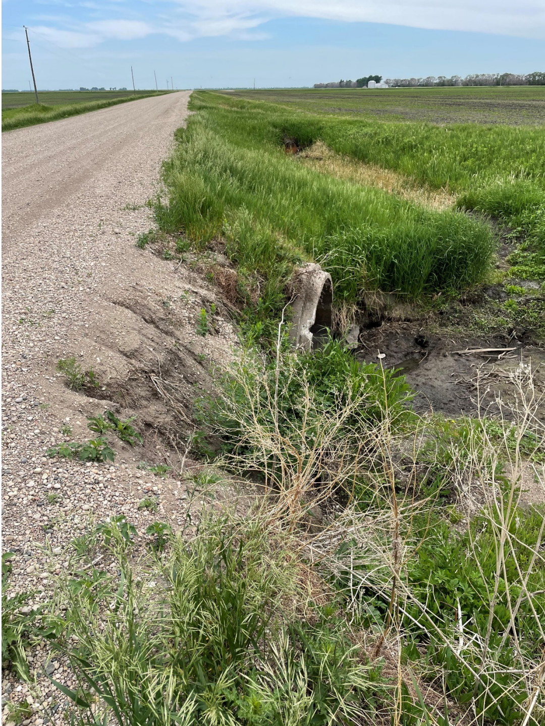
Plugged culvert and road washout along 290 th Ave SW.
