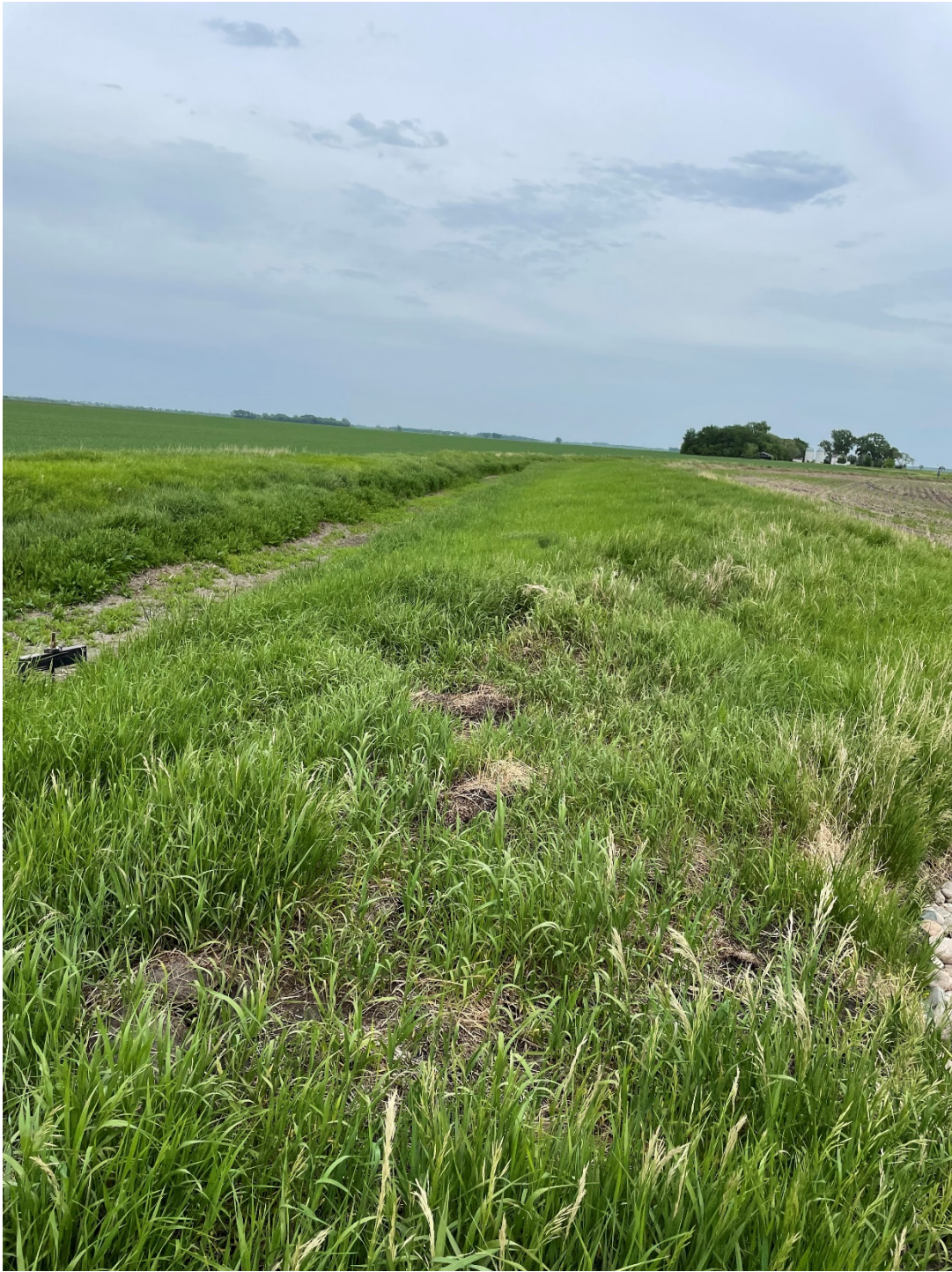
Example of a side water inlet with a screw gate located around station 53+00.
