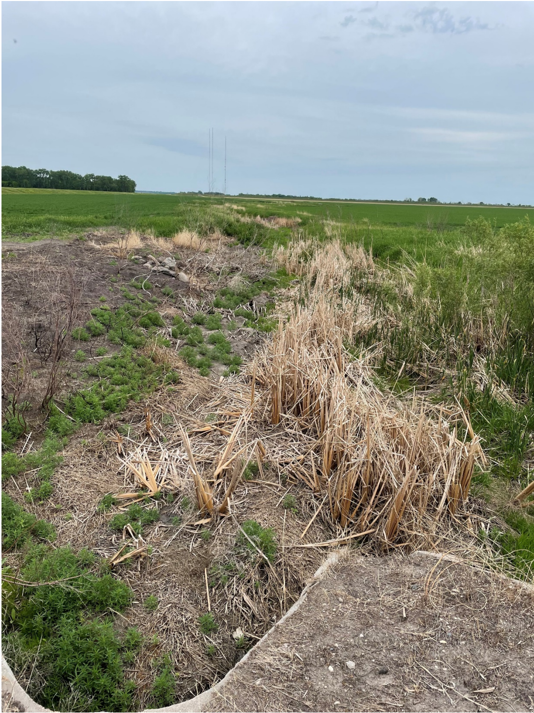
Plugged culvert and poor condition of ditch looking east at 270 th Ave SW.
