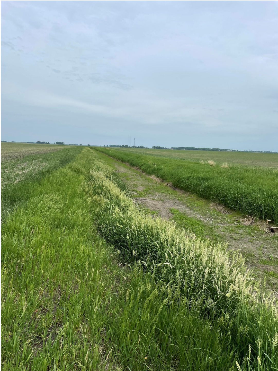
Example of a well-maintained ditch bottom with nicely vegetated side slopes.
